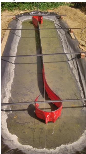
Figure 39. (top) One of the two electrical motors (Model AG 10 1,0M). (bottom) Open tanks for microalgae cultivation. Beginning of works. (right) Scaled pond built before the definitive one was ready in the plant.
