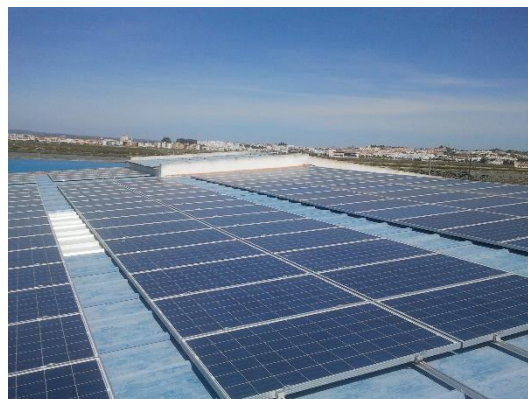
Figure 1. AQUASEF PV panels installed
