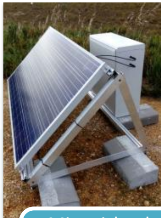
Micro island PV systems 5 x 200W units
