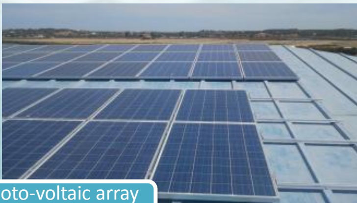
Micro island PV systems 5 x 200W units
